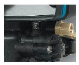
Step 8: Salt Tank Overflow (this is the elbow on the side of your salt tank). Attach 1/2" i.d. plastic tubing to the fitting from the salt tank and run to a drain. This drain line will not be under pressure. DO NOT tie into the backwash drain line! This line should be higher than your drain line. Overflow drain line must be a separate line from fitting to the floor-drain, sewer, tub, etc.
